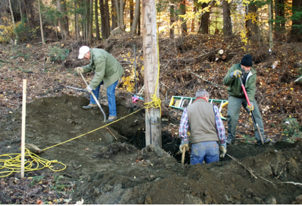
▲ Ascutney Mountain, West Windsor Volunteers building a rope tow for a community ski area on conserved land.
