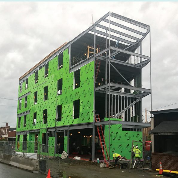
▲ With a $500,000 federal HOME Program loan through VHCB, Railroad Row, LCC is completing 17 new energy efficient apartments in downtown Hartford, to be managed by the Vermont State Housing Authority.
